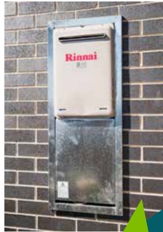
Gas hot water unit.
