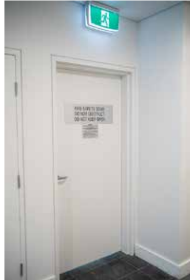
Fire stairs on each level.
