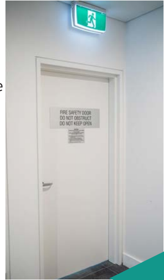
Fire stairs on each level.
